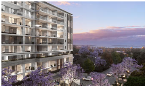
15 Bay Street, Rockdale
